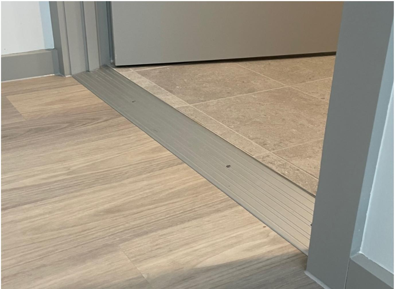
Figure 5.3 Example of a level threshold through the doorway
